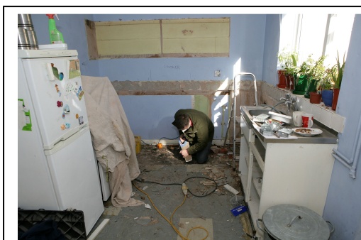
Image 9.1 A Council home before a renovated kitchen is installed.
